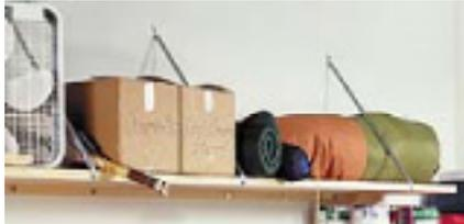
The shelf is made by cutting a standard hollow-core interior door in half. You can make two shelves out of one door. If you don't have a spare door lying around, you can buy one for about \$20.
